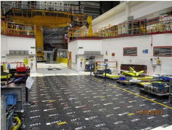
Pile Cap measurement location
