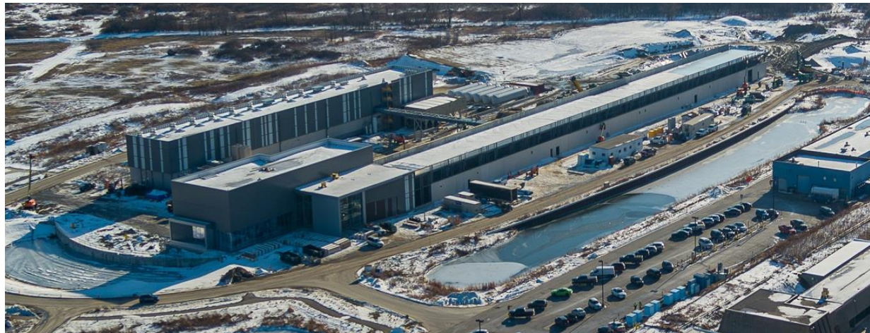
The PIP-II buildings
