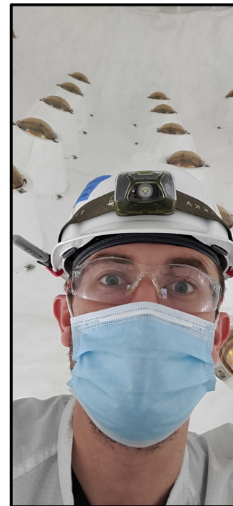
Harvey working on OCS and OD PMT installation.
